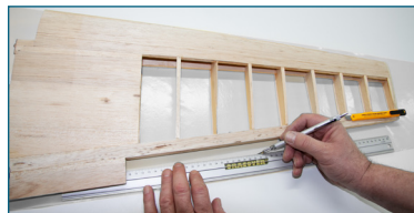
Fig. 12a: Trimming from the aileron recesses
